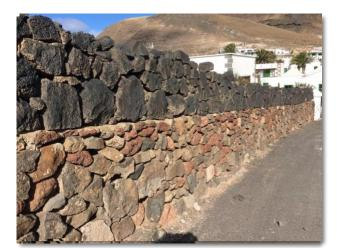
Dry stone walls on Lanzarote are made from the island's natural lava rock quarried from a lava field. The splitting of the rock is done by hand using a diamond-tipped blade in an angle grinder to cut small grooves in the stone in which are placed steel wedges. These wedges are hit with a heavy club hammer and the rock is split. The process is repeated until the desired size of rock is reached.
