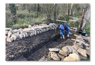
Dave came up with an ingenious method of using stone to insert the words 'Tyneham Farm' into the wall, and he and Tush spent hours trimming stone to create the letters which will be stabilized into the wall using concealed lime mortar. Tush and I got chatting to a retired waller who happened to be visiting and who sold us two new Pennine hammers at a knock down price (pardon the pun).
