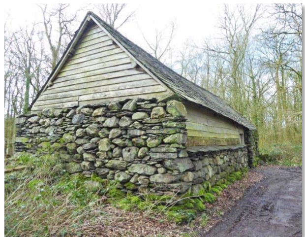
This barn has slate uprights supporting the roof as well as the dry stone shelter.
