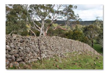
Some of the most outstanding walls are north west of Melbourne, around the township of Buninyong (photo left, DSWAA). The stone comes from the volcanic activity of Mount Buninyong and is relatively small and uniform in size. Consequently, the walls are wider and lower than many other dry stone walls and generally not coped.
