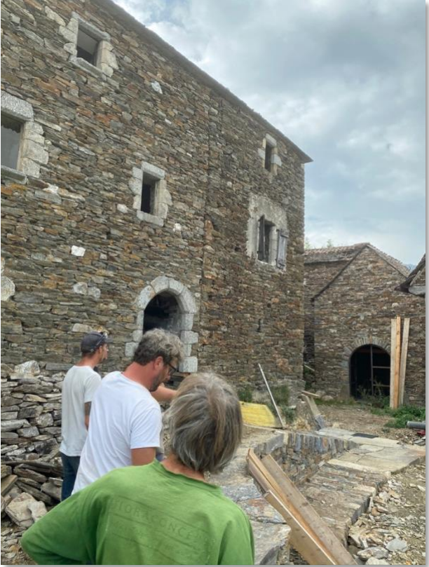
Constructing a drystone house (right) and a close-up (below) of a perfect arched doorway
