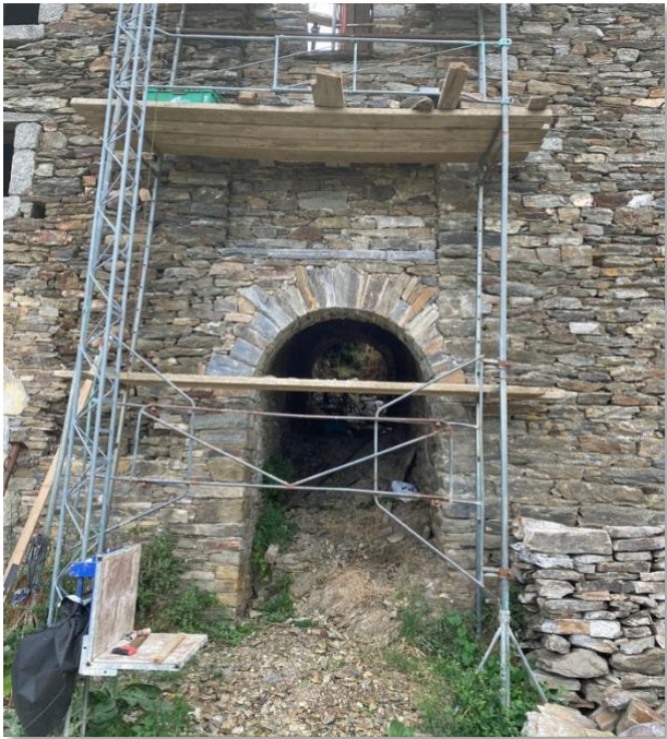
Constructing a drystone house (right) and a close-up (below) of a perfect arched doorway
