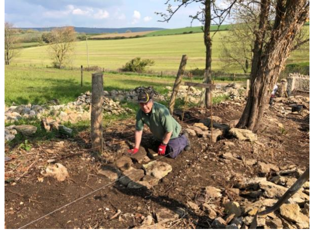
Phyllis and Wendy clear the last of the old foundation stones while Geoff lays the first footings of his section of wall. Strings are up, ready to go!
