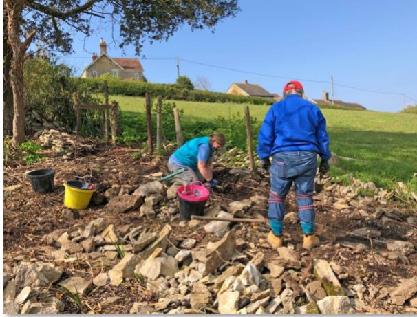
Phyllis and Wendy clear the last of the old foundation stones while Geoff lays the first footings of his section of wall. Strings are up, ready to go!
