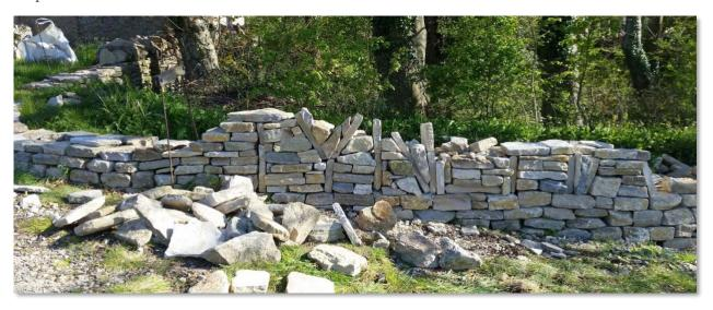
And here's the latest image. This is by no means a straightforward project. Peter says that one of the most difficult parts of the build is finding the right size and shape of stones to butt up against the stones that make the letters. I'm particularly impressed by the triangular stone that fills the top section of the letter 'A' in the word 'Tyneham'.
