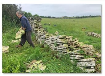
Ian begins to take down the wall and stack the stone. We have decided to take this section down to the foundations because we are uncertain how they have been laid. Dave thinks the wall has been built either on flat foundation stones or by knocking the foundation stones into the ground at the angle of the slope and building up the courses from a sloping basement level.
