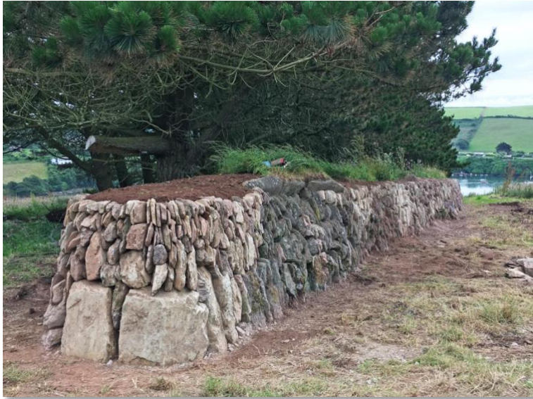
This stunning retaining wall with round quoin end was recently completed by Martin at Bigbury-on-Sea.
