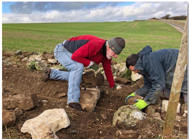
The copes have been cemented onto the wall and take a bit of getting off. Sally resorts to the bar!
