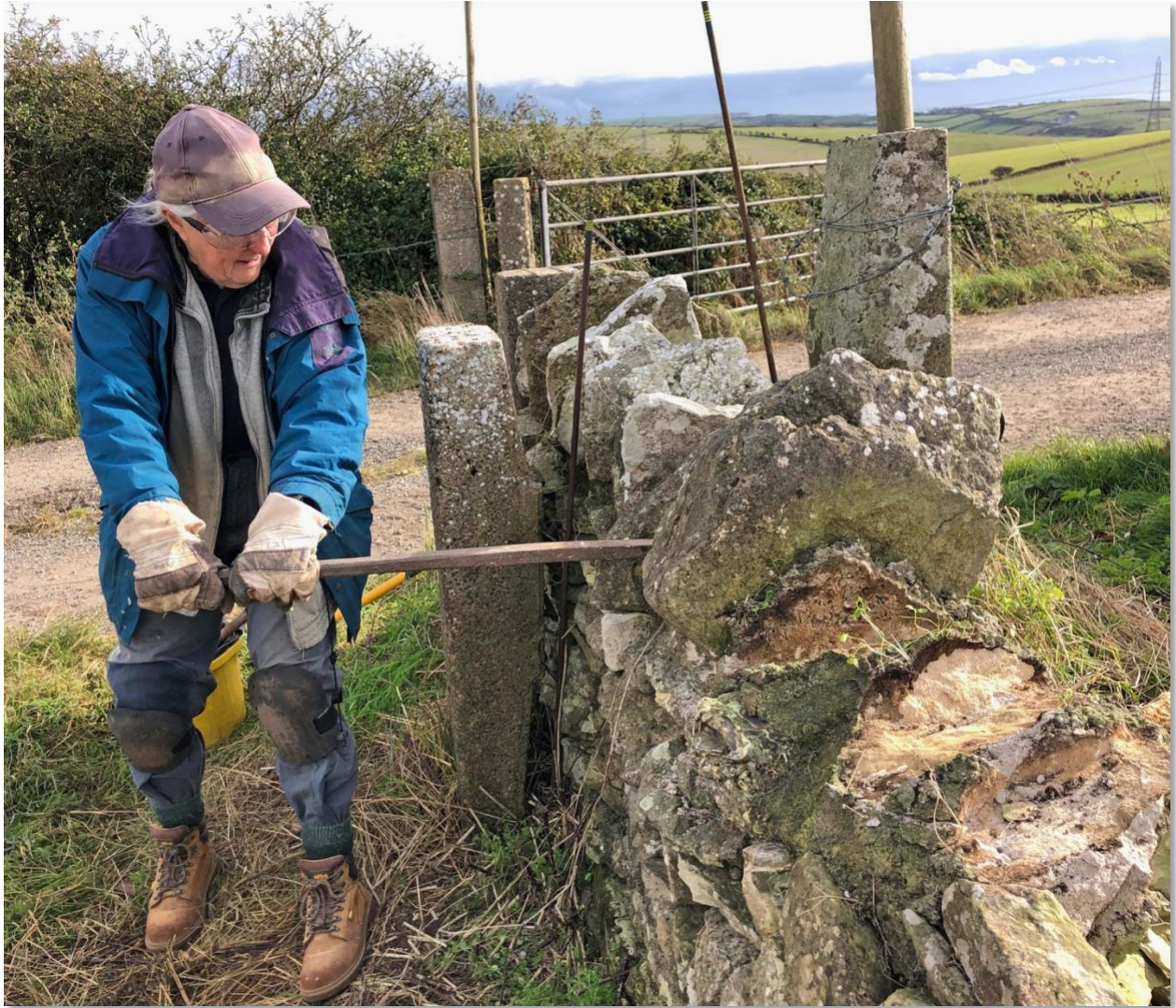
The copes have been cemented onto the wall and take a bit of getting off. Sally resorts to the bar!
