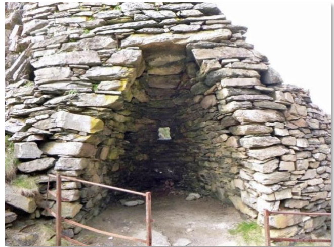
Above: Restored 19 th century limekiln at Heddon's Mouth (more or less on the beach) on Devon's north coast, once a popular venue for smugglers. Note the corbelling of the roof.
