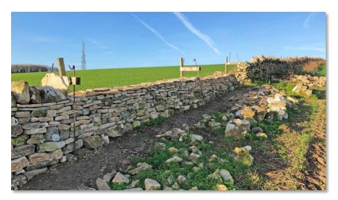
I was the first on site on this sunny but cold morning. There's a section of wall ready for coping, another section to complete, and a new section to be taken down and cleared for foundations. Plenty to keep everyone very busy.
