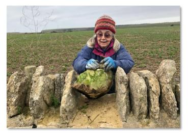
And talking of cemented copes, Wendy circumnavigates the wall picking up fallen copes, scraping off the cement, and re-laying them.
