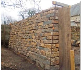
'I am also a recent convert to Jed's trick of securing lines with bulldog clips, rather than fiddly elastic bands and S-hooks. These work really well with Screwfix (other suppliers are available) high visibility builders line, which has enough elasticity to keep the line taught, but enough give to minimise any trip-hazard.'
