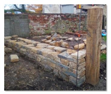
'I had originally intended two rows of through stones, but had very few of sufficient length, and needed these as cheek end ties. Instead, used three-quarter through stones, in Cotswold style, throughout the build. Because of the regularity of the stone, I was able to use a batter of 1/10, rather than the "textbook" 1/8. Anyway, the Dorset style tends towards the vertical.'
