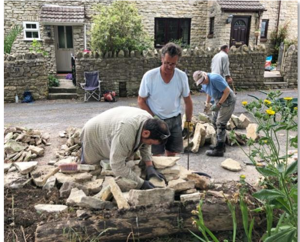
Peter sets up the strings as we all arrive to continue working on this wall.
