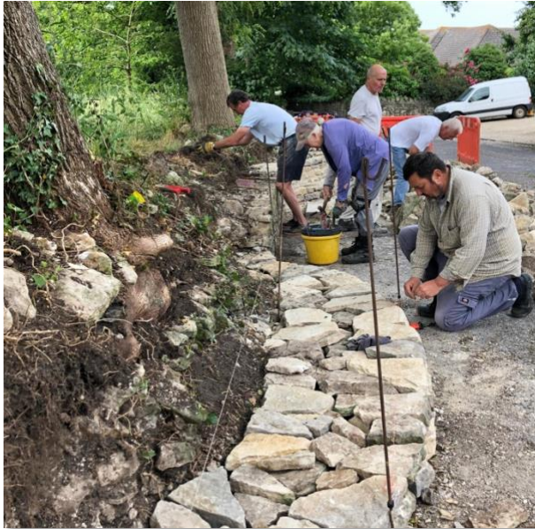
Peter sets up the strings as we all arrive to continue working on this wall.
