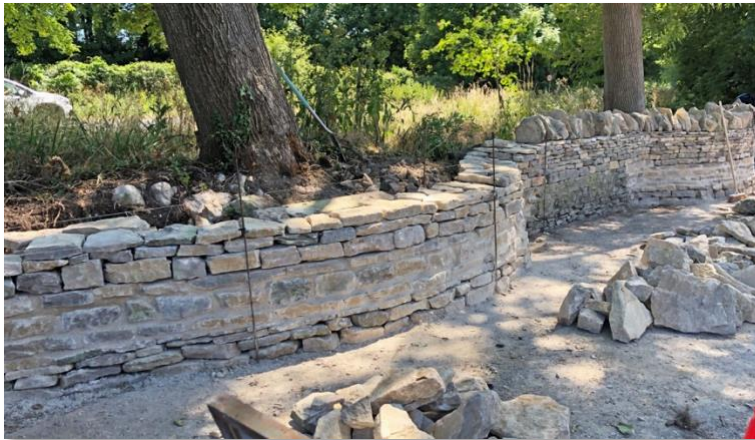
Phyllis and Mary cope a completed section of wall.
