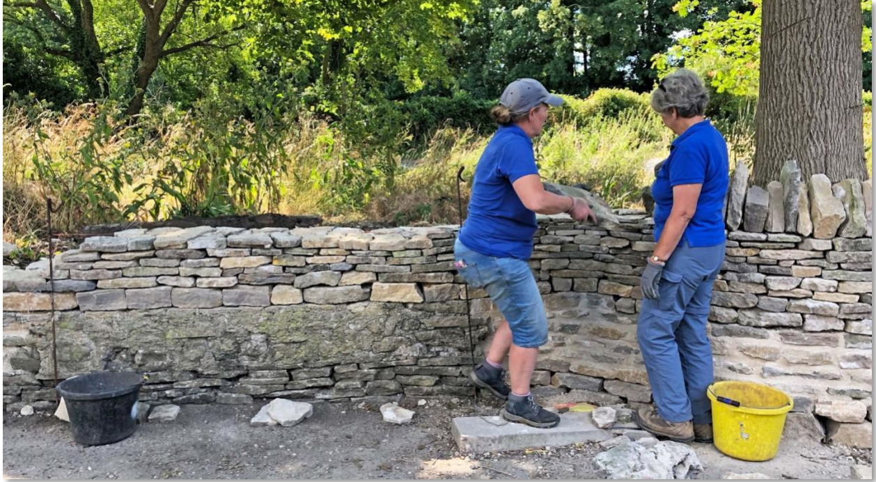
Phyllis and Mary cope a completed section of wall.
