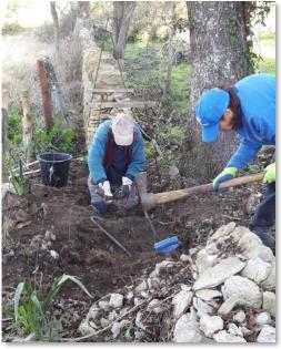
By mid-afternoon, however, we have cleared a good section of the wall, dug out a foundation trench, and Sally has laid the first foundation stones.
