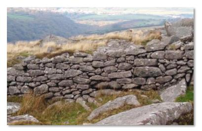
The Dartmoor walls are built with huge boulders - in some the gaps are filled (probably from the front!) with small pieces of stone but in others (below) they are left with the holes. This is supposed to deter sheep from climbing over.
