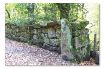
Sally recently spent a walking weekend on Dartmoor and photographed these dry-stone structures. An impressive cheek-end near the River Teign between Fingle Bridge and Castle Drogo. It is the boundary of an old deer park note the copes oversailing the top to discourage them from jumping out.
