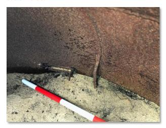
The turret could be rotated through a full 360 degrees and the photo left, which I took inside an Allan-Williams gun turret on Studland, shows the handle used to pull the turret around on its metal wheel cut into a groove.
