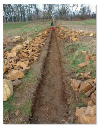
Geoff and his wallers make good progress preparing the foundation trench for their next section of wall ... and find a tiny ammonite.
