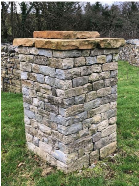
Example of a square pillar built for the Master Craftsman qualification.
