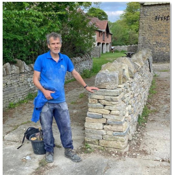
Left: Tim building his first cheek end ... and below: the finished wall.
