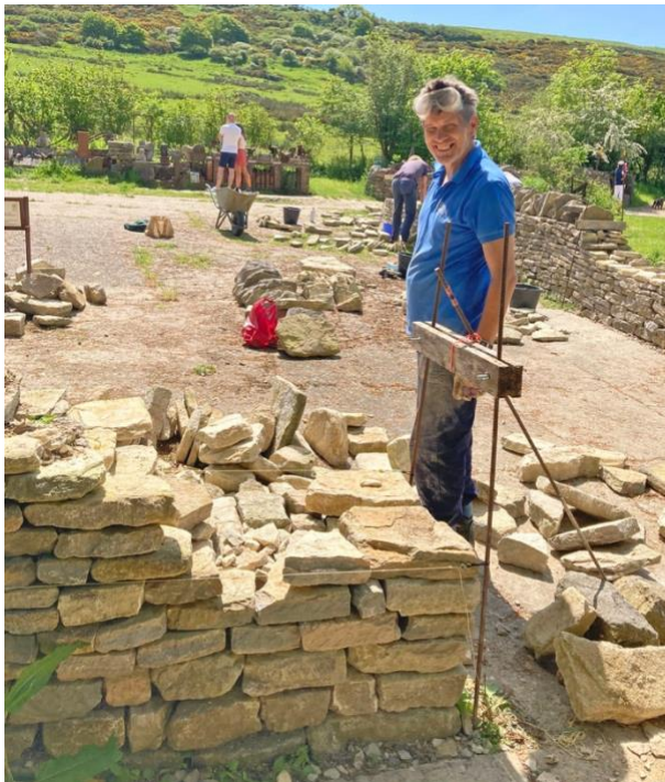
Left: Tim building his first cheek end ... and below: the finished wall.
