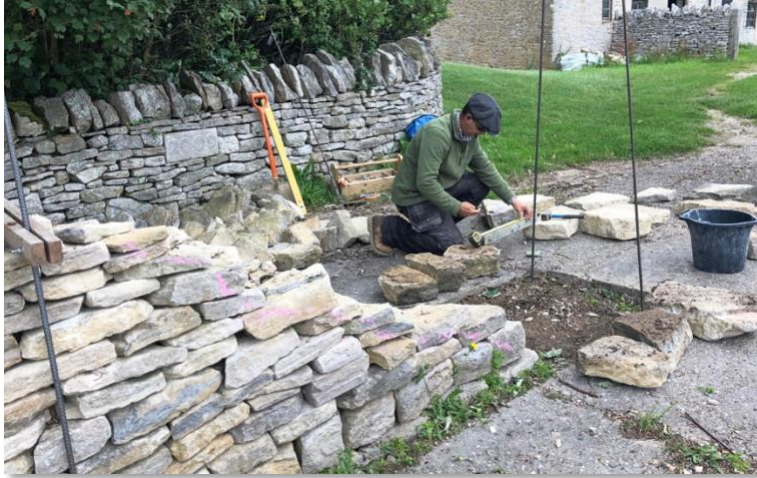
Steve measures and checks the level of his foundation stones.
