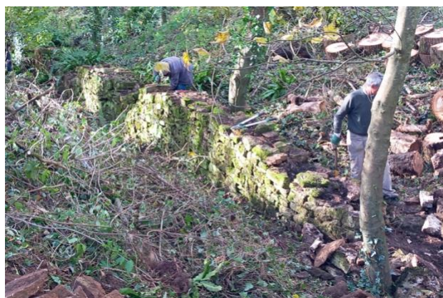
Walling on the rampart section and restoring the wall junction on the ramparts.
