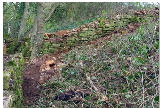
Walling on the rampart section and restoring the wall junction on the ramparts.
