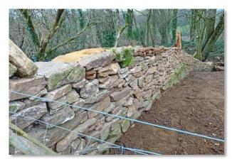
In late February, Geoff wrote: 'This week, we will continue with restoring the c.400-year-old parish boundary wall in the rampart ditch. Given that we have 50 metres of copes on order, and the wall up the ramparts is c.15 m, we can aim to get about 35 m of boundary wall up to height. It should be a bright day, if a little chilly and claggy underfoot (understatement Geoff although it looks a lot drier at Ham Hill than it does at Corton or Purbeck.)
