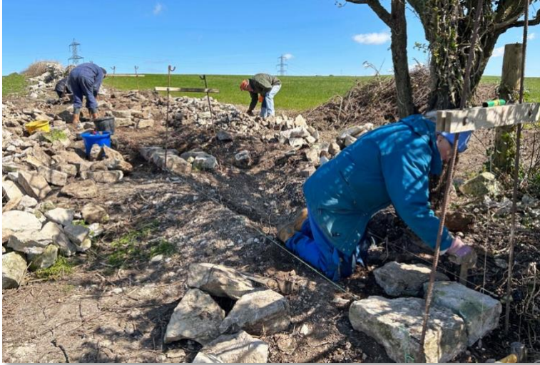
Heads down in the search for foundation stones. Adrian and Tush pick up stone while Sally makes a start on the cheek end.
