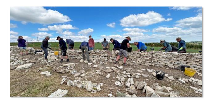
It's back to full sun now and the second lift is well underway. Through stones have been placed into the wall at regular intervals. At Corton, we tended to keep the stints separate but building a complete wall by both teams makes for a much nicer finish and more interest for the participants.
