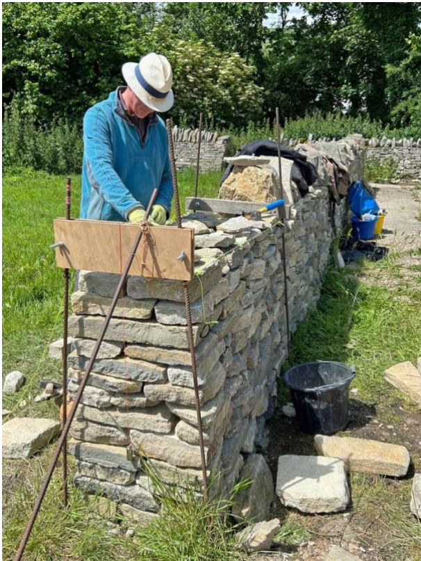
Peter advises on setting up the batter frame for a cheek end.
