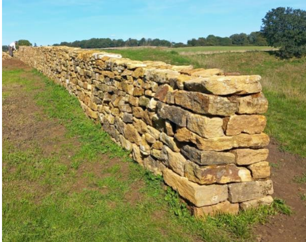
The completed section of wall on Butchers Hill with Geoff's trademark chunky cheek end!
