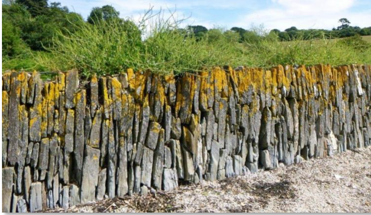
Left and below: Lovely vertical walling on a retaining wall at the back of Trelissick Beach, a National Trust site near Truro.
