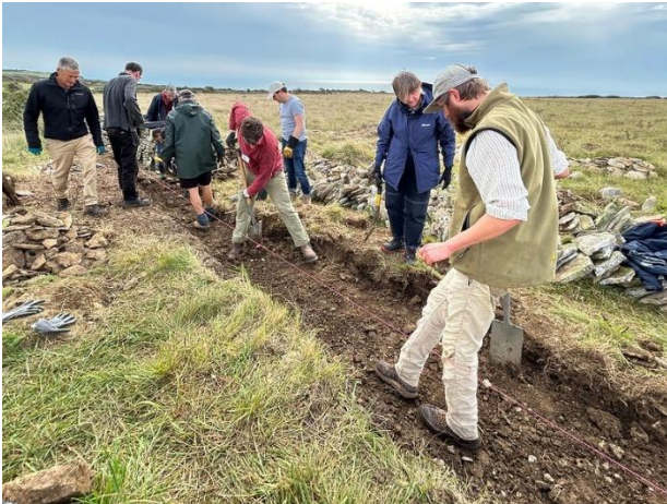
Foundation trench being prepared in the sunshine in the morning
